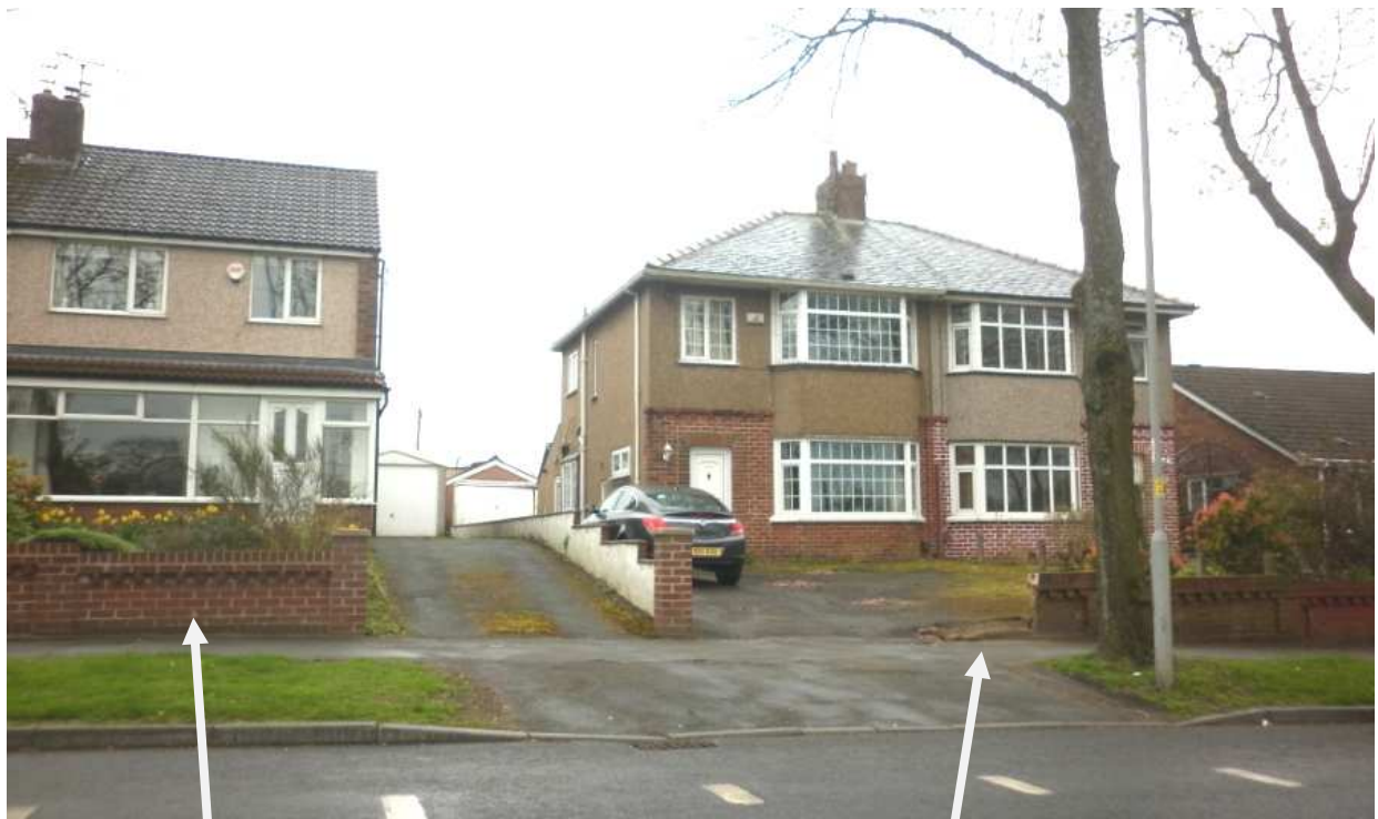
no.59 no.57 Windermere Ave – part of garden wall removed
