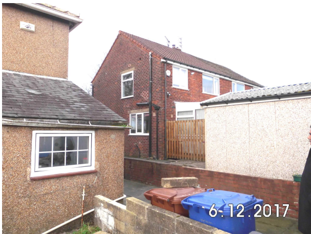
looking towards the rear of no.59
