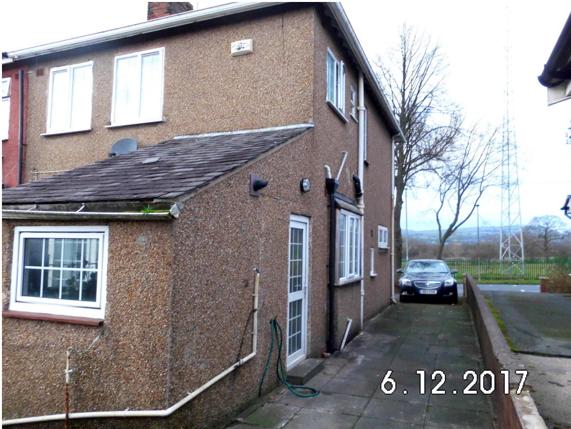
existing rear/side of no.57 Windermere Ave
