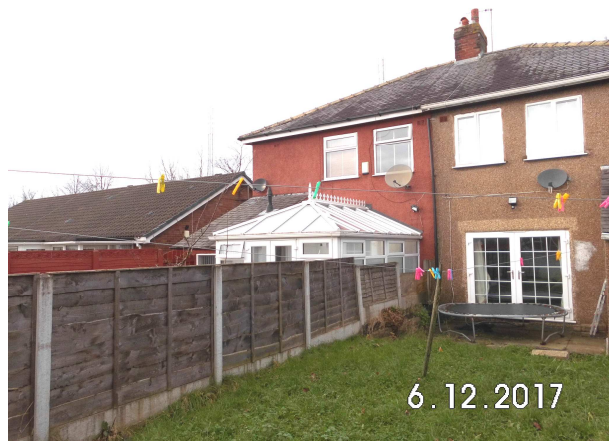
looking towards the rear of no.55
